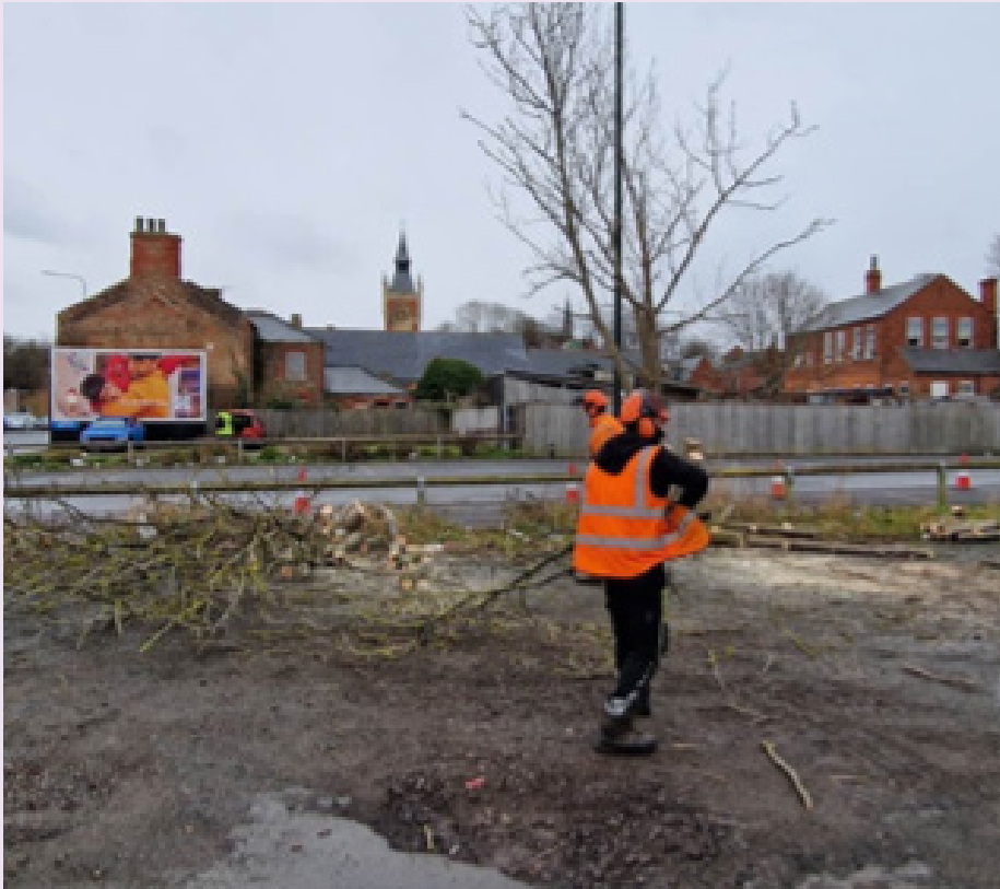
Wellington Street Car Park - removed wild trees and overgrown foliage prior to new permanent CCTV installation (high-risk VAWG area). Three new lighting installations, and new lampposts supporting the new CCTV network.
